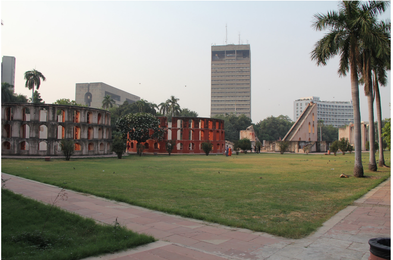
Figure 22 : Overall View of the Complex
