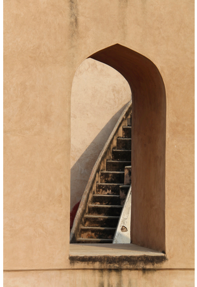
Figure 1 : View of the side stairs of the Samrat Yantra
